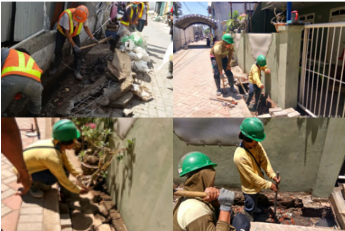
Perbaikan saluran untuk jalan warga di kawasan Vasa Hotel Surabaya dan Voza Premium Office Drainage renovation for the society at Vasa Hotel Surabaya and Voza Premium Office area, Surabaya
